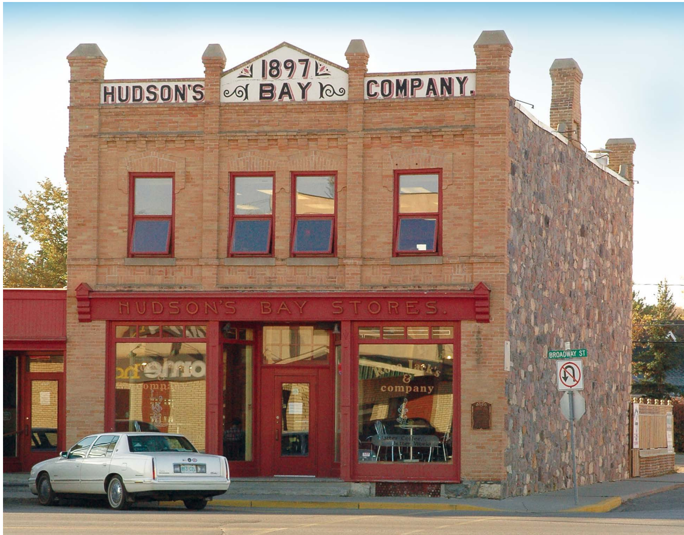
Above: View of the north-facing brick façade and west wall constructed of fieldstone. Photo: C. Fehr
