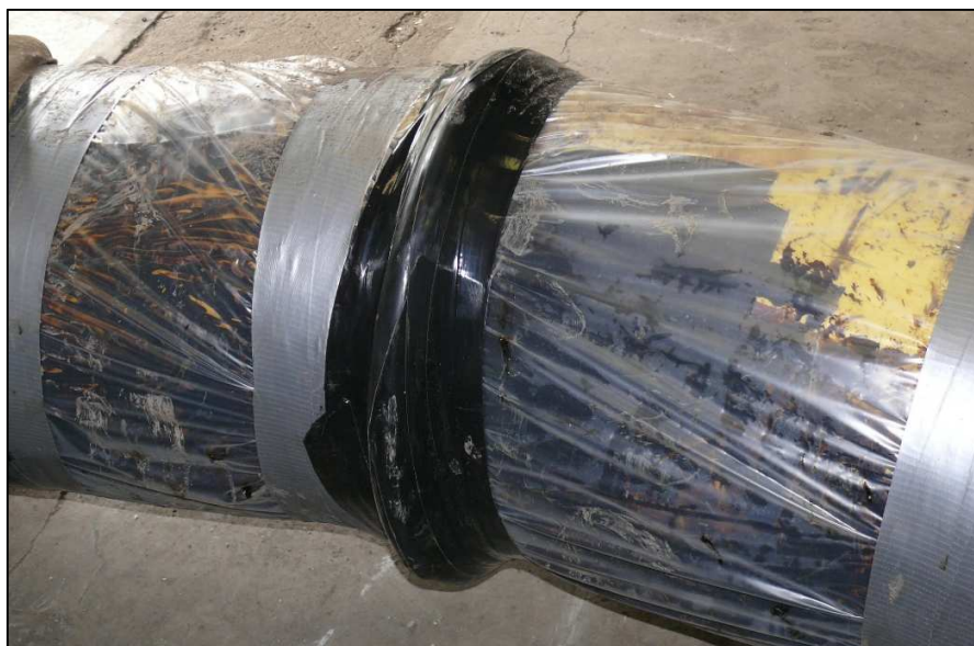
FIGURE 4 AS-RECEIVED TAPE AND PLASTIC WRAPPING ON FAILED BUCKLE ZONE
