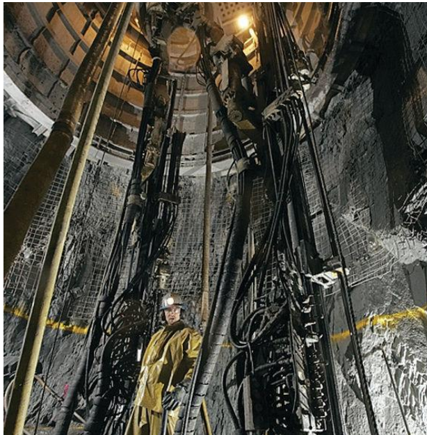
Figure 9:2 Shaft sinking in progress
