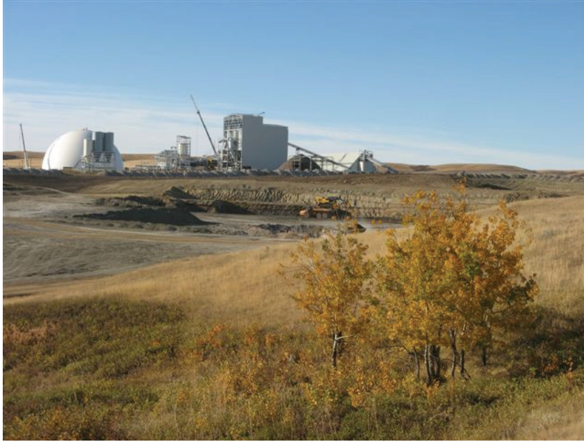
Figure 14 - Gollier Creek Mine of Whitemud Resources Inc., looking southwest across the initial overburden excavation in the West Pit towards the processing plant. Primary crusher is on the right; product storage dome and loadout on the left. Photo courtesy of Ron Olchowski.
