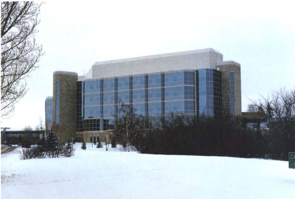
The recently built Agriculture Building at the University of Saskatchewan featuring dolomite from the Deschambault Lake area.
