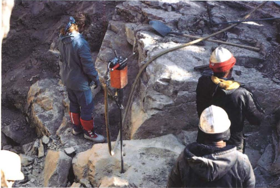
Dolomite evaluation and development at Deschambault Lake.
