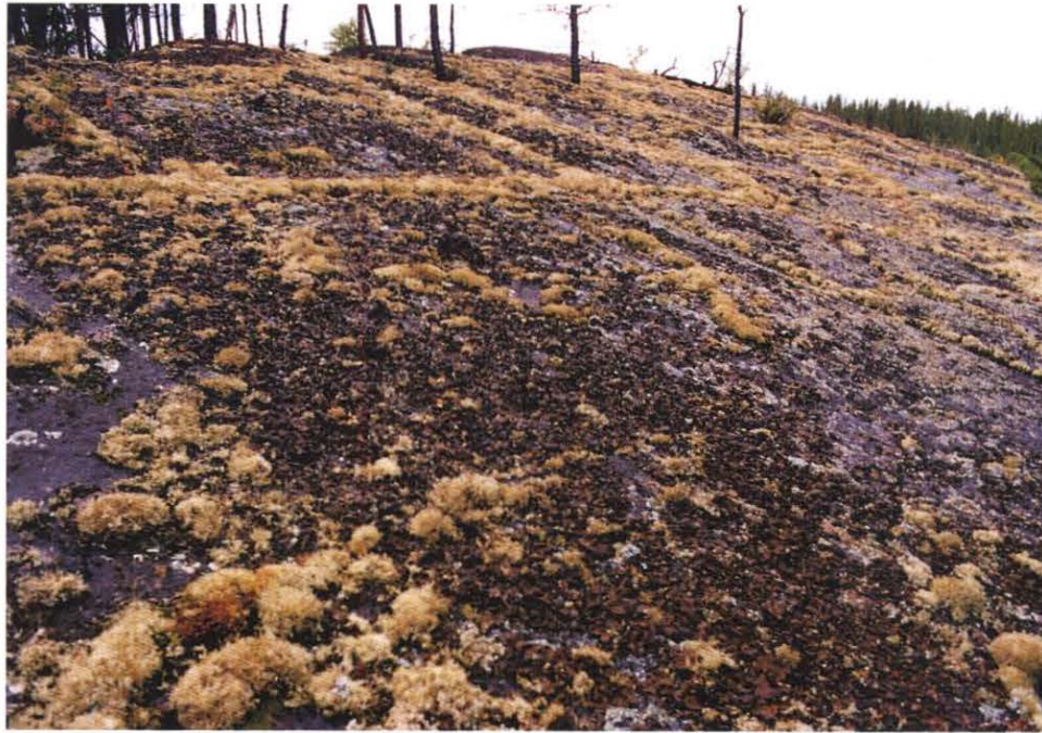
Lichens delineate the wide spacing of fractures in this stone.
