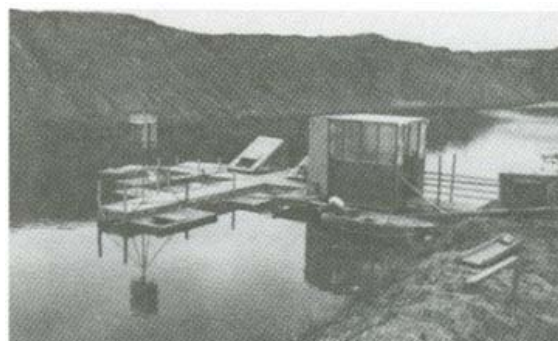
An example of fingerling holding facilities in Saskatchewan.
