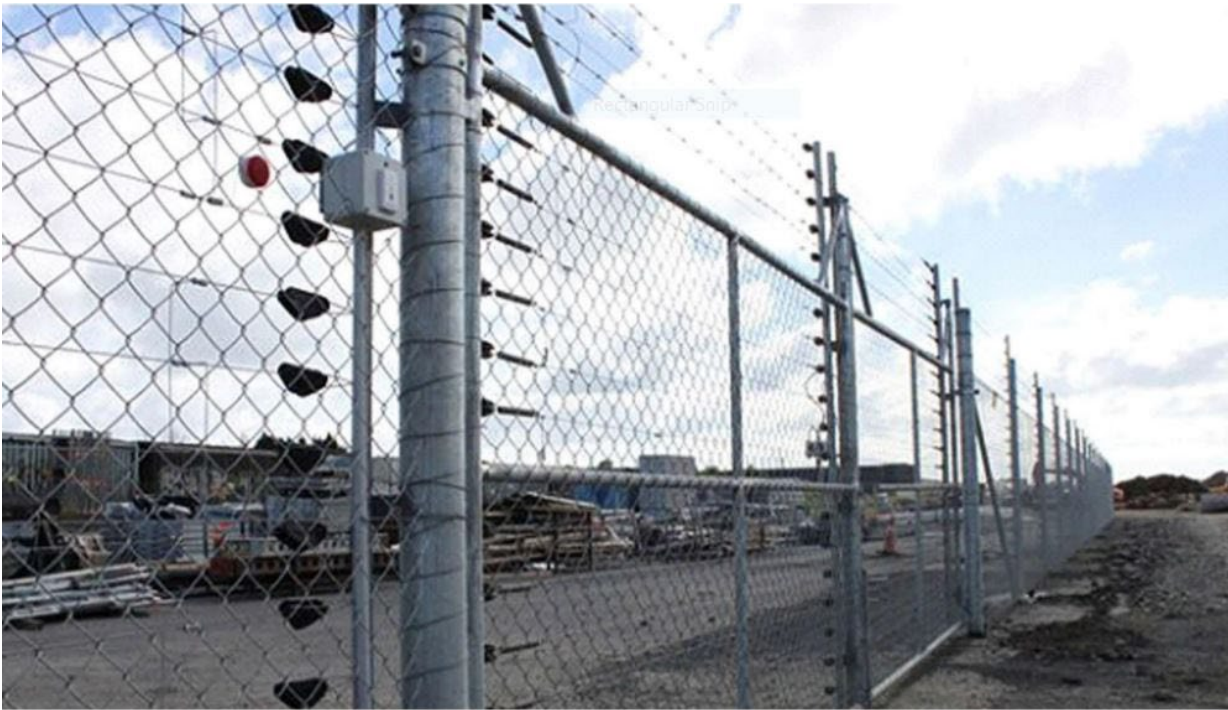
Chain link and electrified fence example ( skweldedmesh.com/electric-fence/ )
