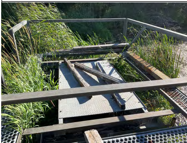
Image 3. Water control structure (location #5 on Figure 3-2) with overgrown vegetation choking the structure and preventing proper function.
