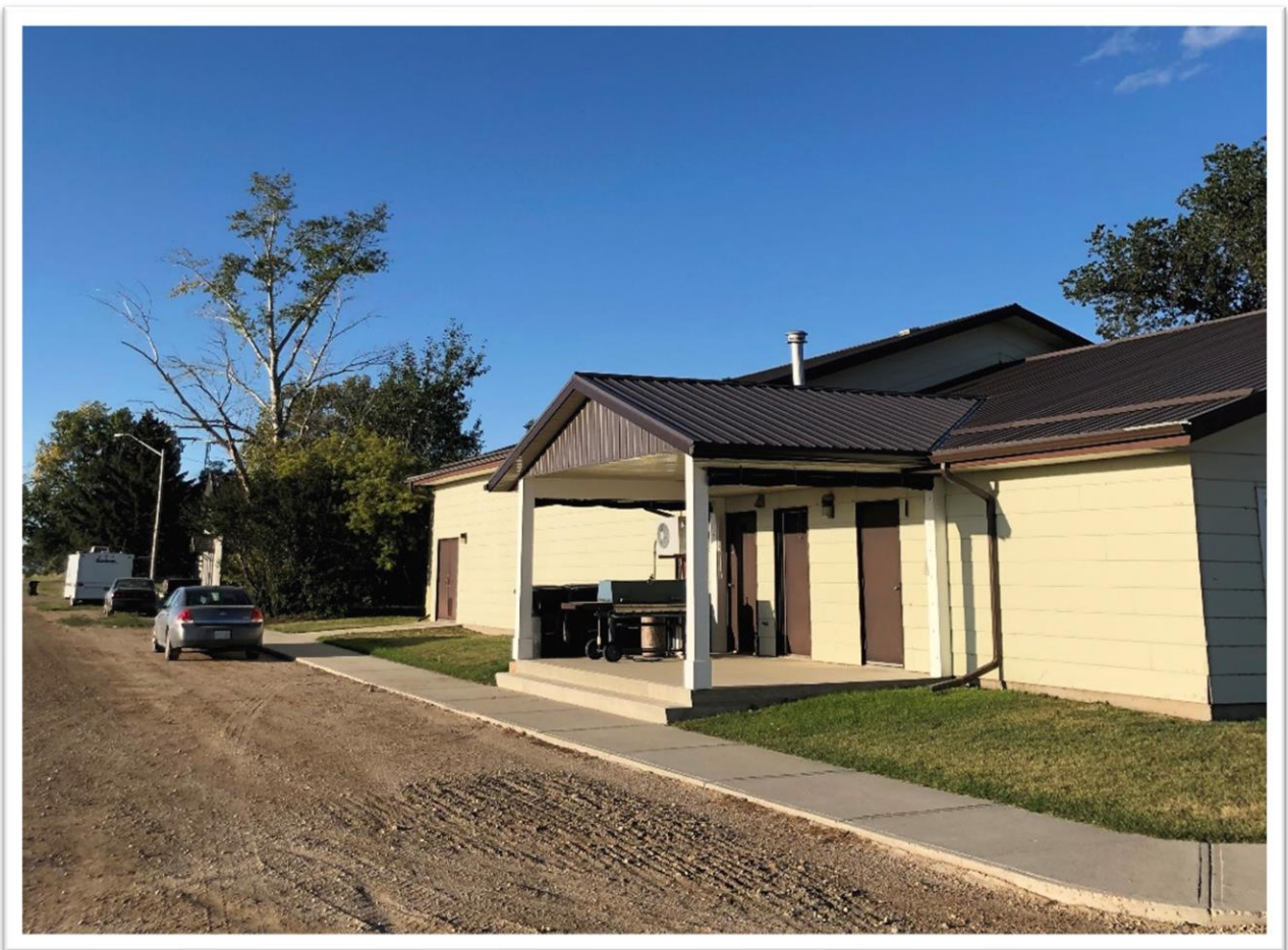
Duval Hall Wind Shelter (Photo Courtesy: Village of Duval)
