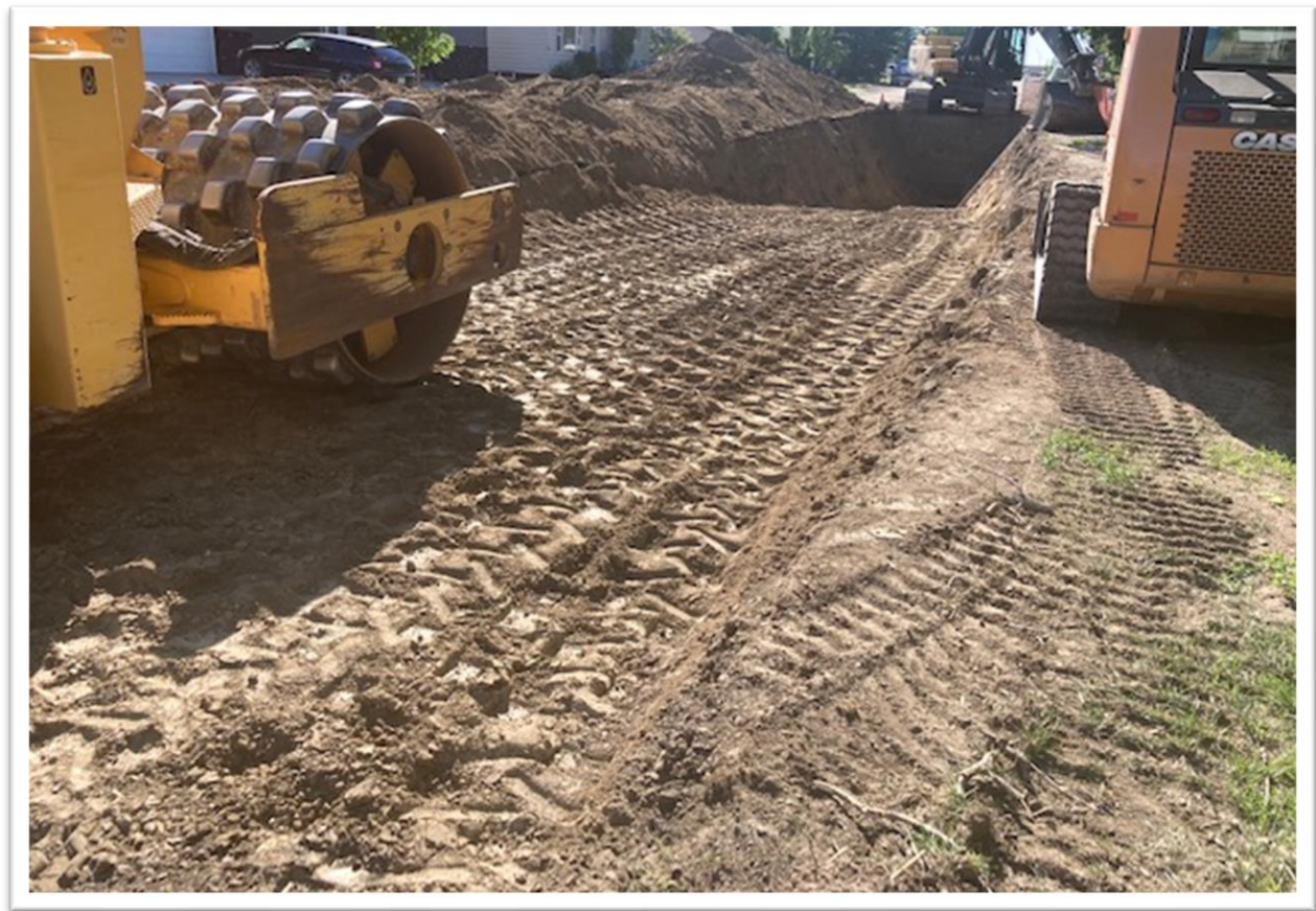
Replacement of 180 metres of sewer line, two manholes and 12 connections (Photo Courtesy: Town of Hague)
