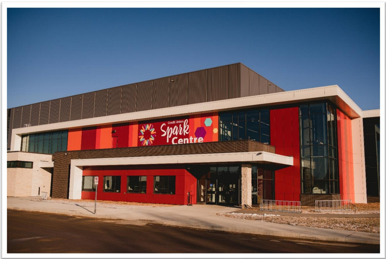
Weyburn Recreation and Cultural Centre (Photo Courtesy: City of Weyburn)
