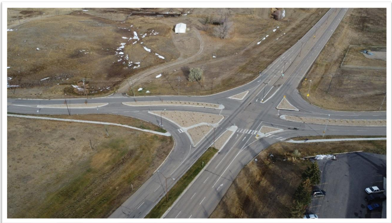
Re-alignment of Battleford Trail and Central Avenue Intersection (Photo Courtesy: City of Swift Current)
