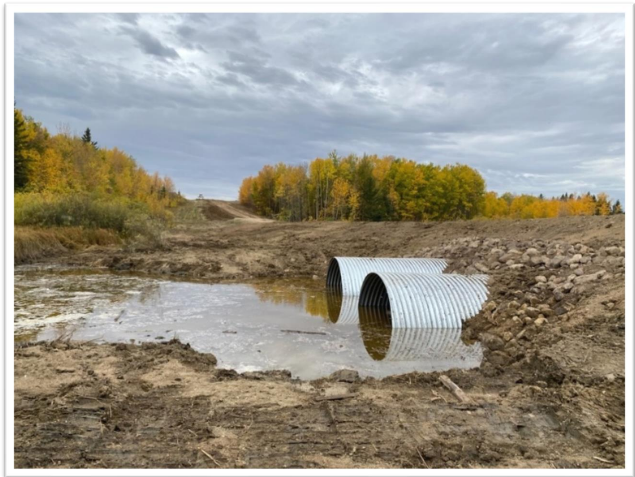
Replacement of two steel culverts (Photo Courtesy: Rural Municipality of Arborfield No. 456)
