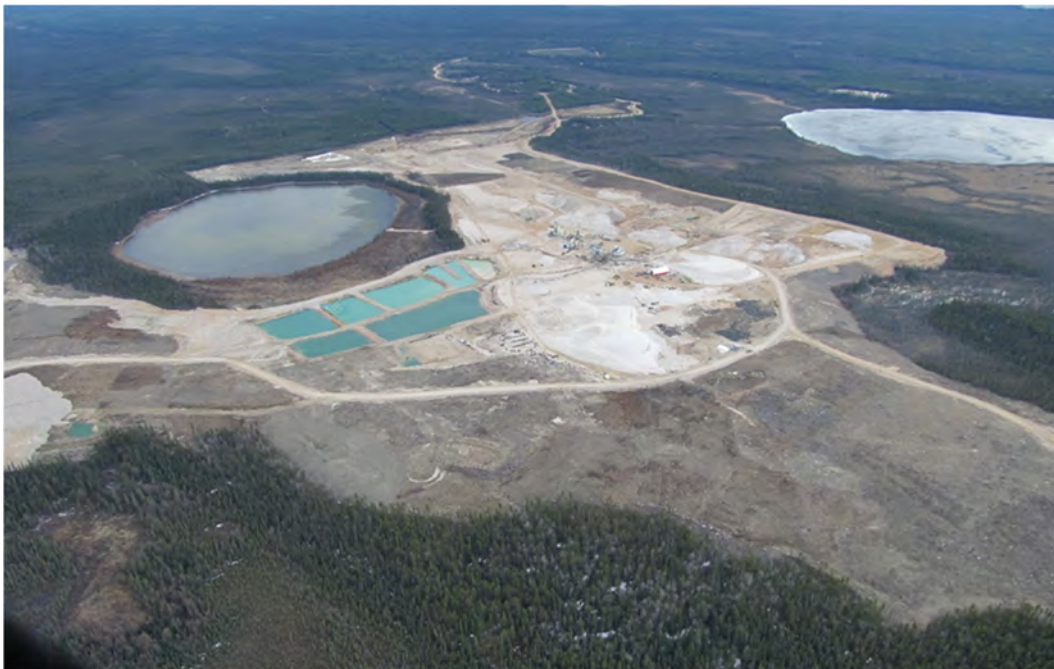
Figure 3-3 Hanson Lake Facility during Operations in 2012
