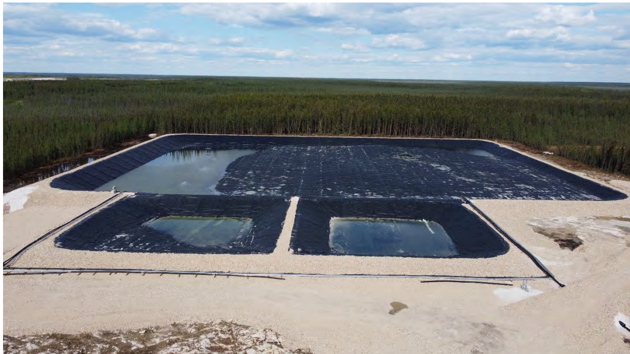
Figure 3-38 Image of Constructed Effluent Storage Pond
