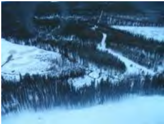
Cigar Lake Tie In Looking West
