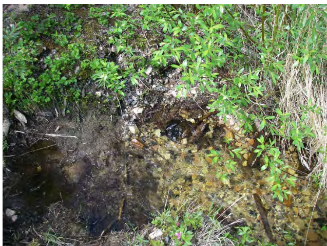
Photo 11. Location where stream emerges from subsurface approximately 100 m downstream from crossing (2010)
