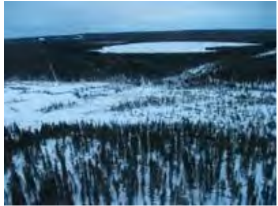
Power Line - Near km 48.4
