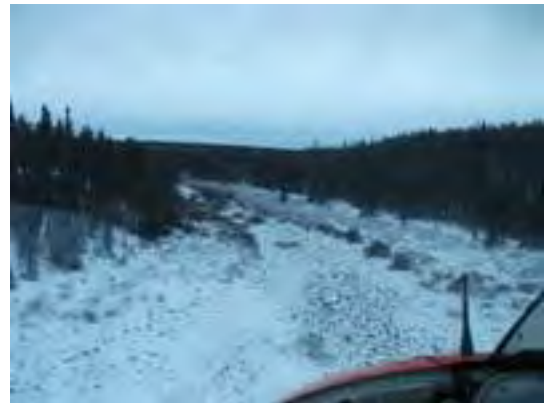
Old Drainage Channel – Near km 31.5
