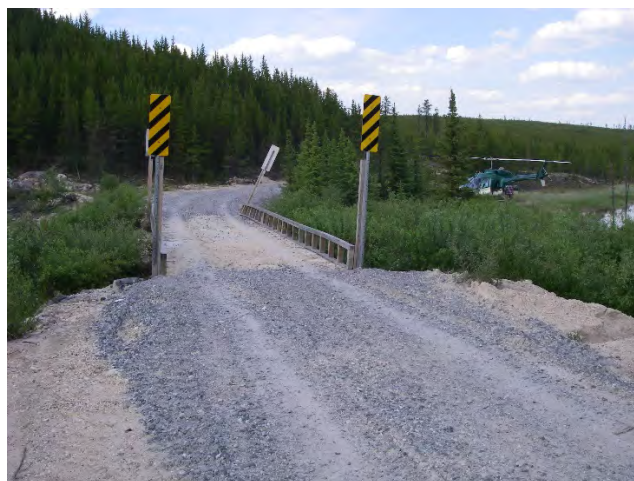
Photo 12. Existing crossing at crossing at crossing (2010)
