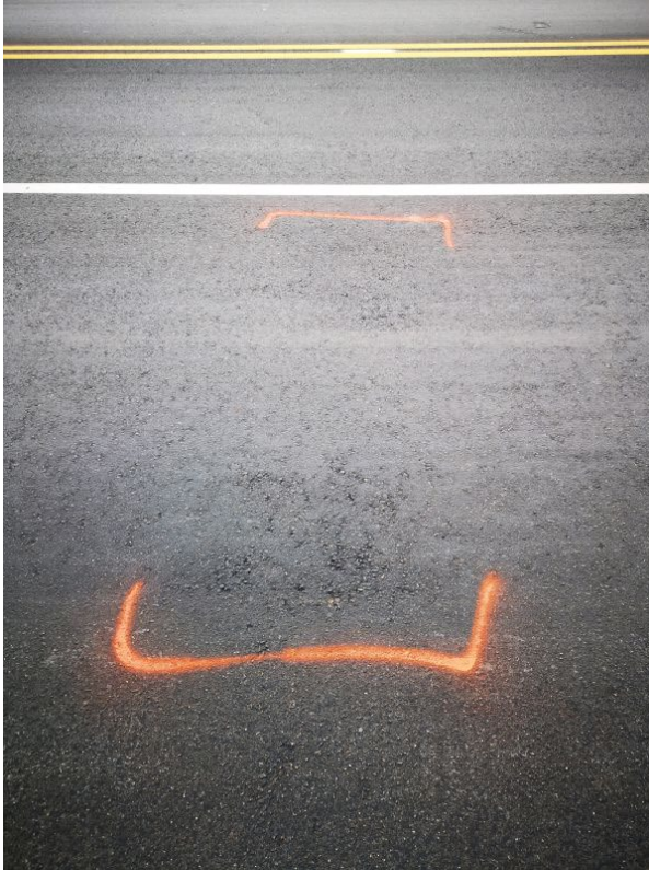
Figure 2: Slight Segregation
