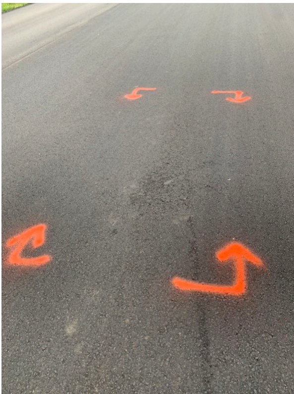
Figure 6: Slight Segregation
