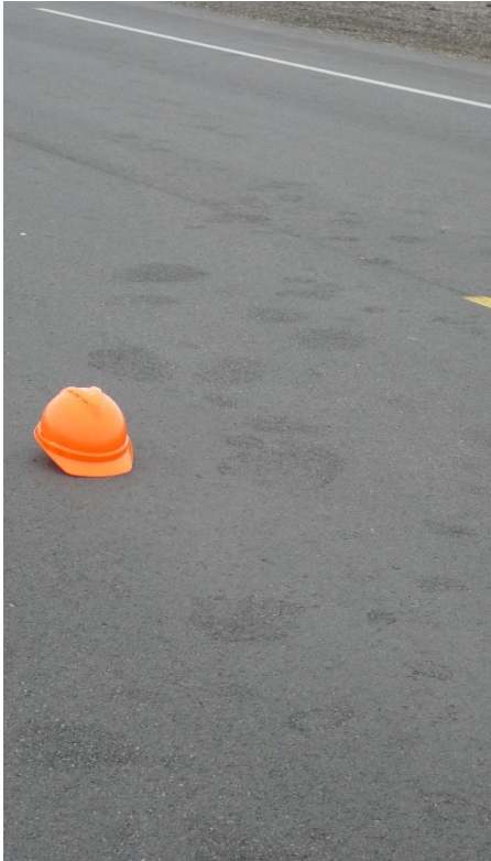
Figure 42: Contaminant Leaks on Surface
