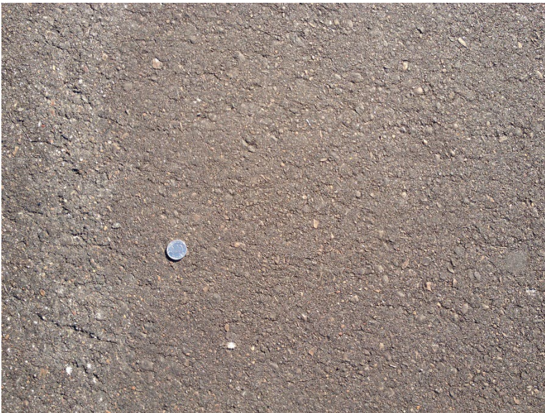
Figure 43: Contaminant Leaks on Surface
