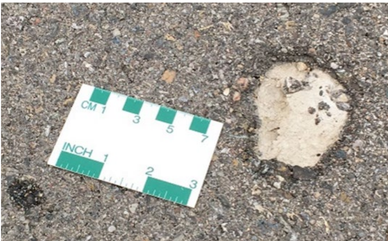
Figure 46: Inclusion of Lime Clump
