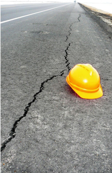
Figure 32: Longitudinal Cracking
