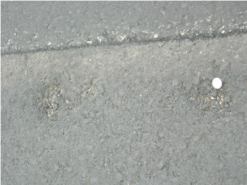
Figure 48: Surface Contaminated With Aggregate
