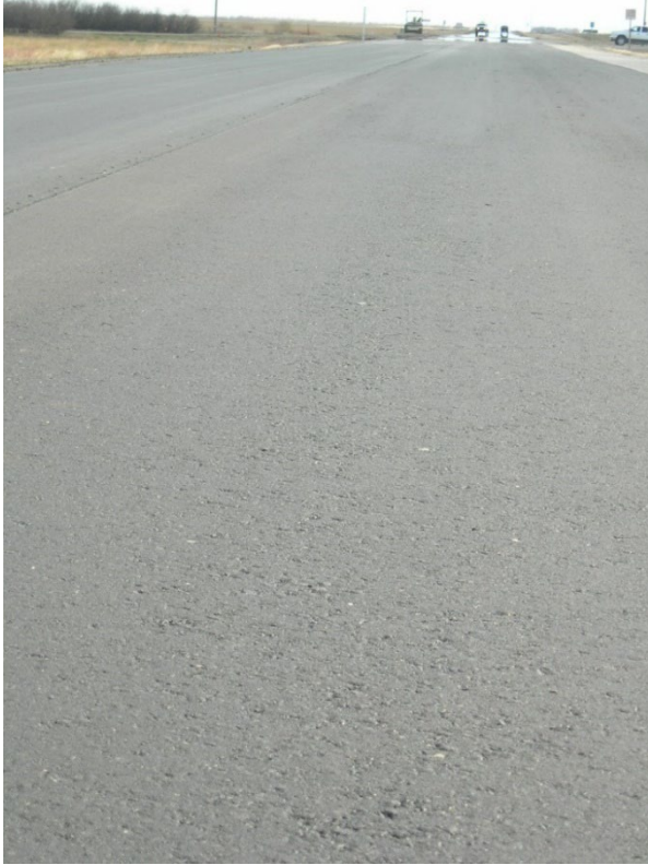
Figure 7: Slight Segregation
