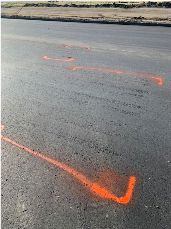
Figure 24: Pneumatic Tire Pick-up
