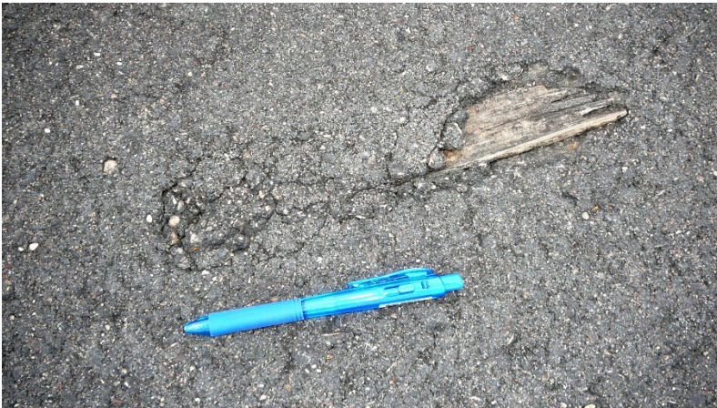
Figure 50: Inclusion of Foreign Object
