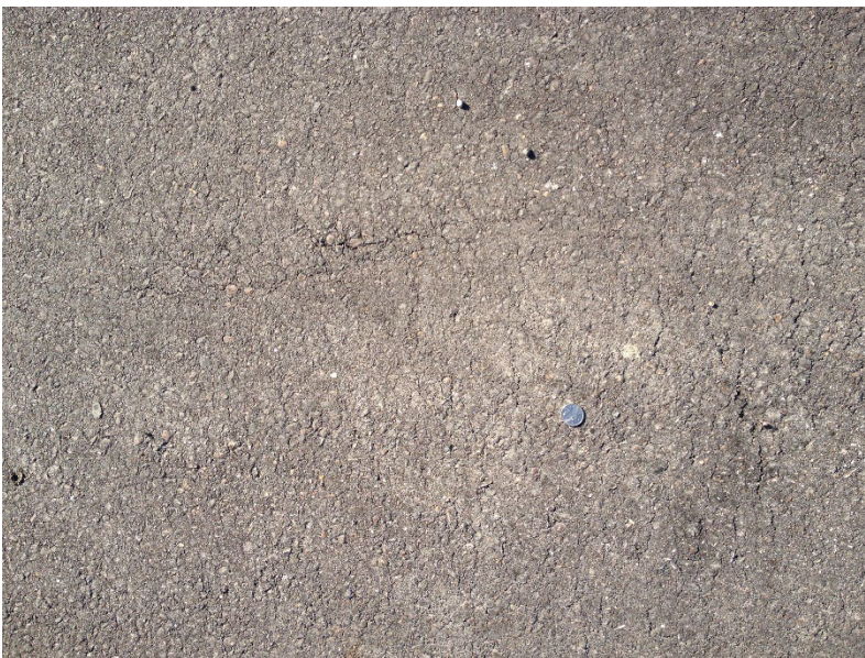
Figure 34: Micro-cracking
