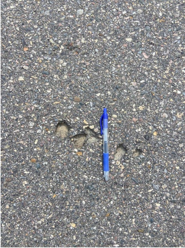
Figure 41: Multi-Stone Pick-Out
