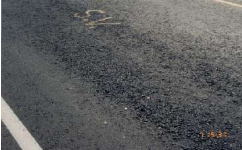
Figure 12: Severe Segregation
