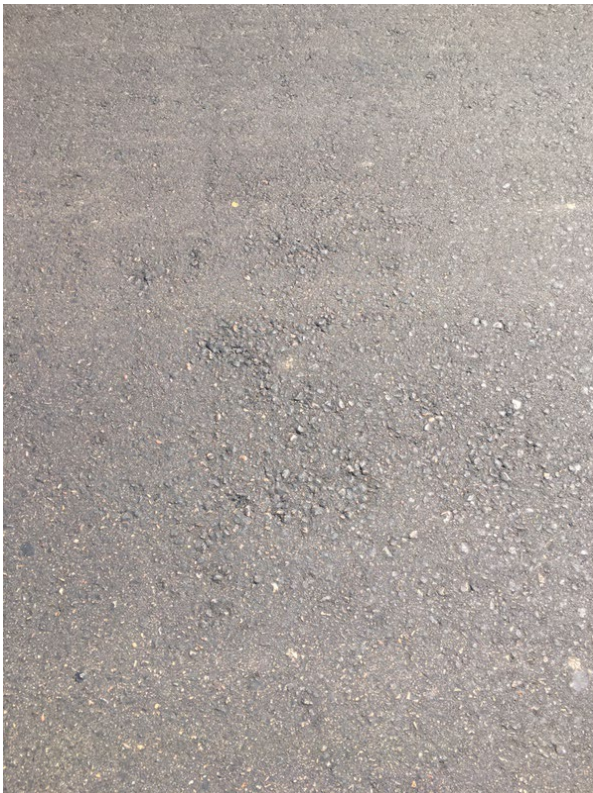
Figure 8: Slight Segregation
