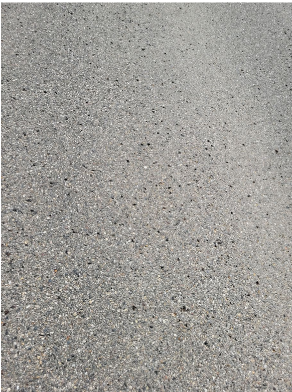
Figure 40: Single-Stone Pick-Outs
