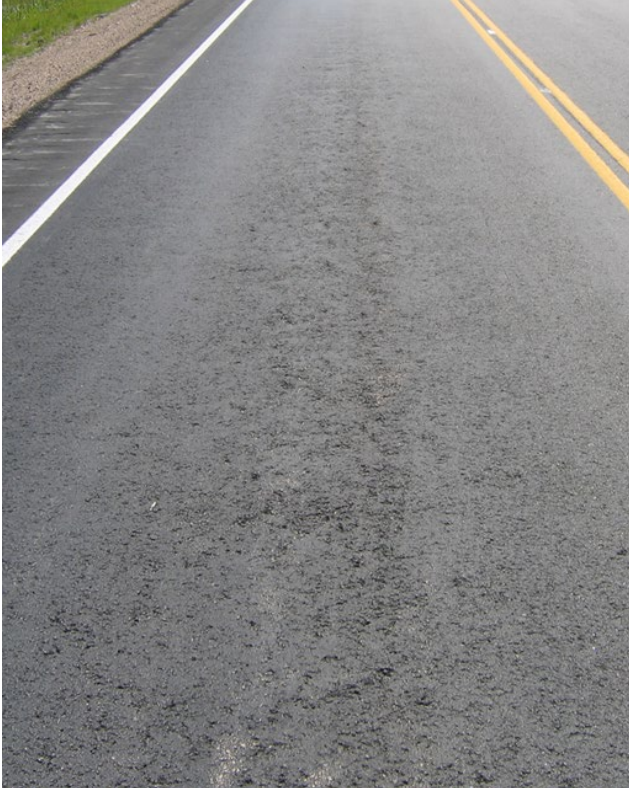
Figure 36: Tearing
