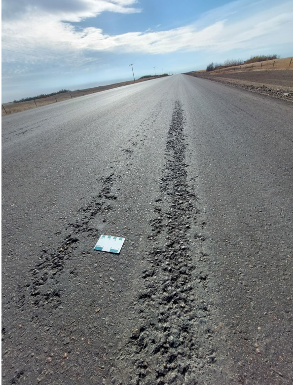
Figure 25: Pneumatic Tire Pick-up
