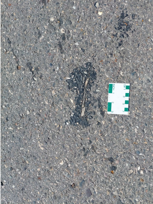
Figure 51: Inclusion of Tree Root
