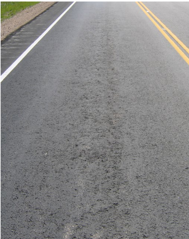
Figure 11: Moderate Segregation
