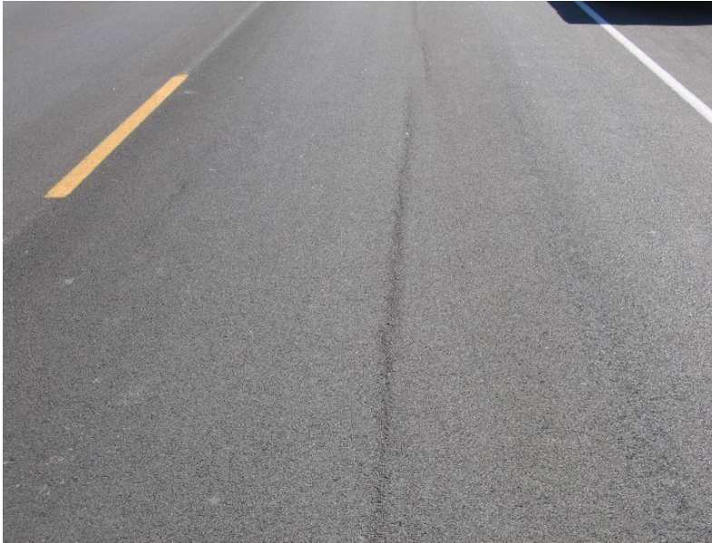
Figure 23: Longitudinal Roller Mark, Tearing/Discontinuity
