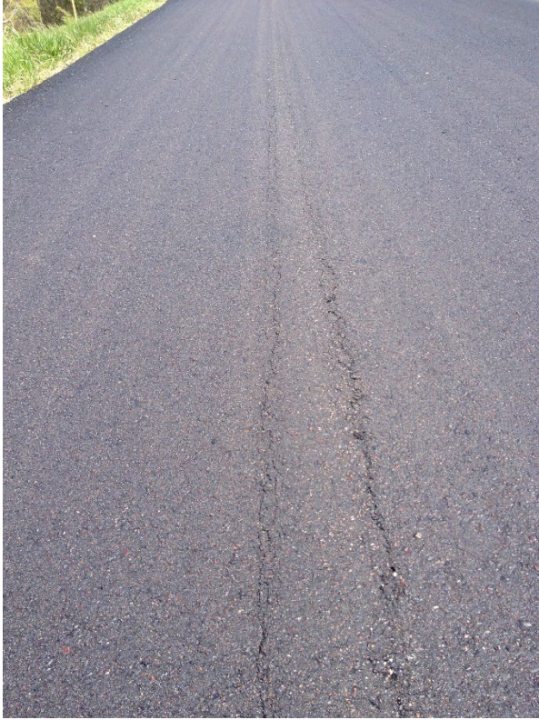
Figure 31: Longitudinal Cracking
