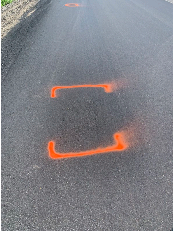
Figure 5: Slight Segregation
