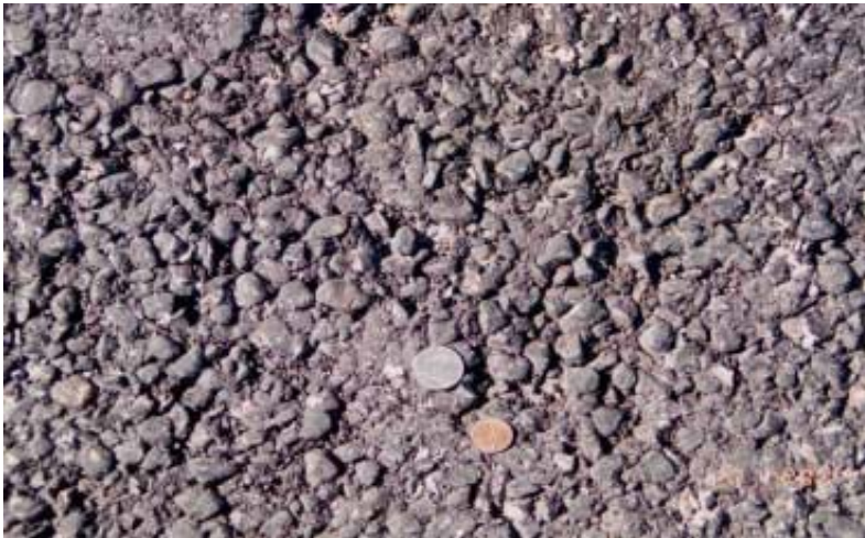
Figure 13: Severe Segregation
