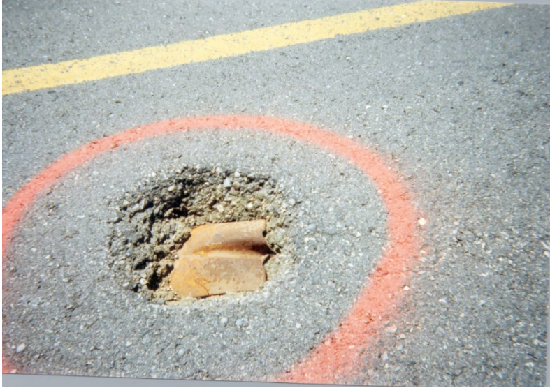
Figure 49: Inclusion of Foreign Object
