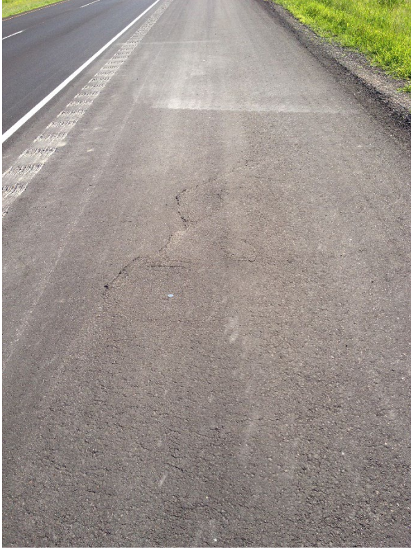
Figure 35: Slip Failure
