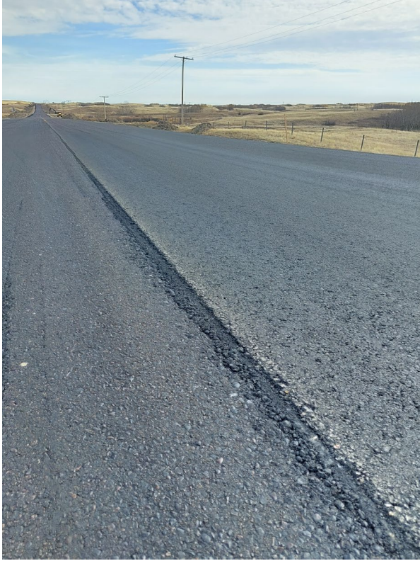
Figure 21: Improper Matching of Longitudinal Joint
