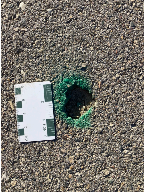
Figure 47: Pothole/Void
