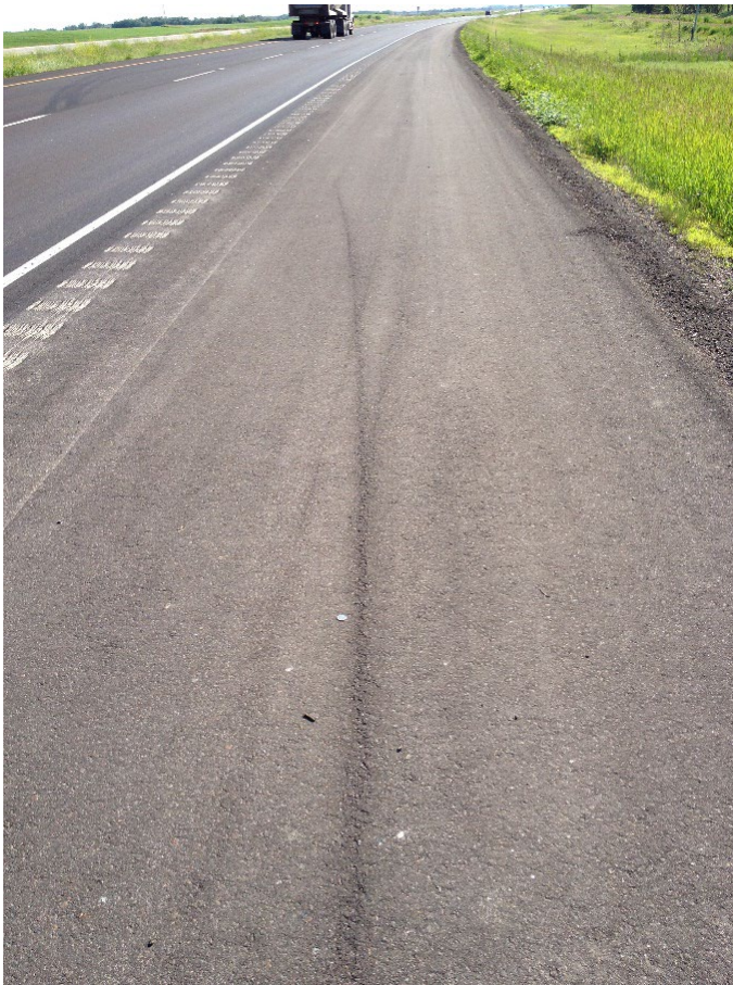
Figure 22: Arc-shaped Roller Mark, Tearing/Discontinuity
