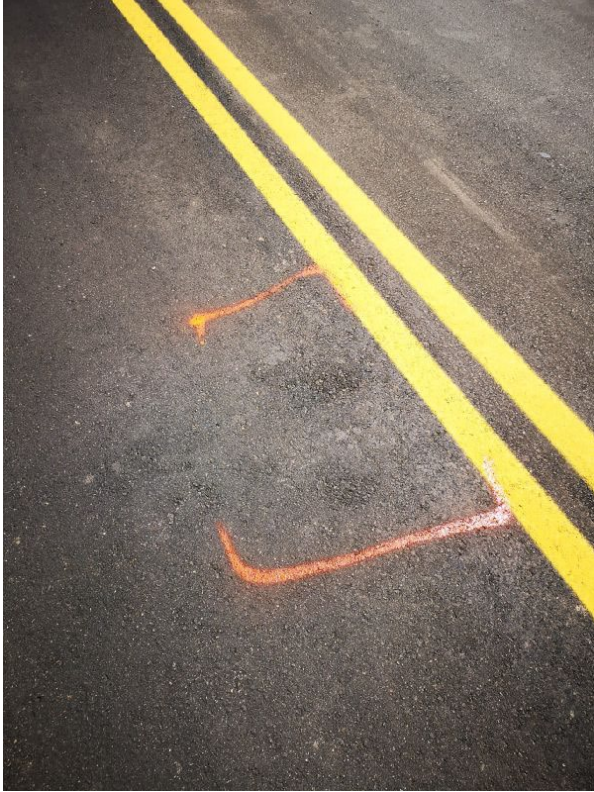
Figure 3: Slight Segregation
