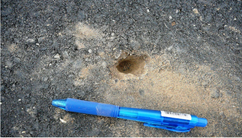
Figure 44: Inclusion of Clay Ball
