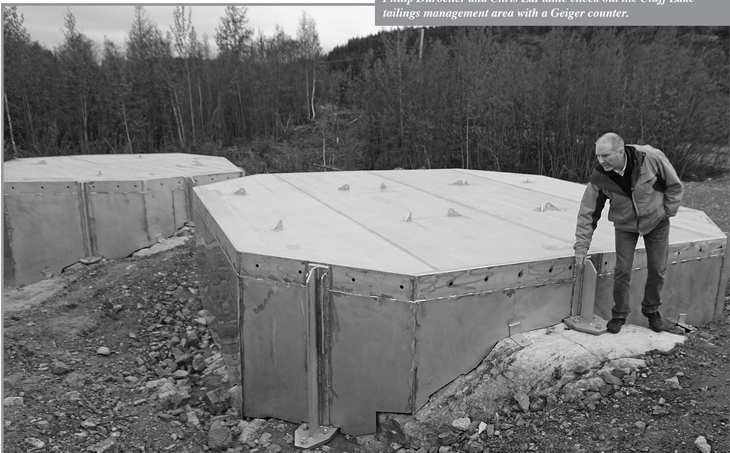
Cameco's Mike Webster checks out the custom-built solid stainless steel covers now securing former mine shaft openings on the Beaverlodge property. The covers are bolted to the bedrock, and include ports where a small camera can be inserted for inspection.
