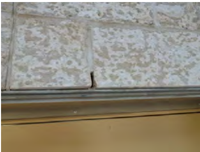
missing weep vent
