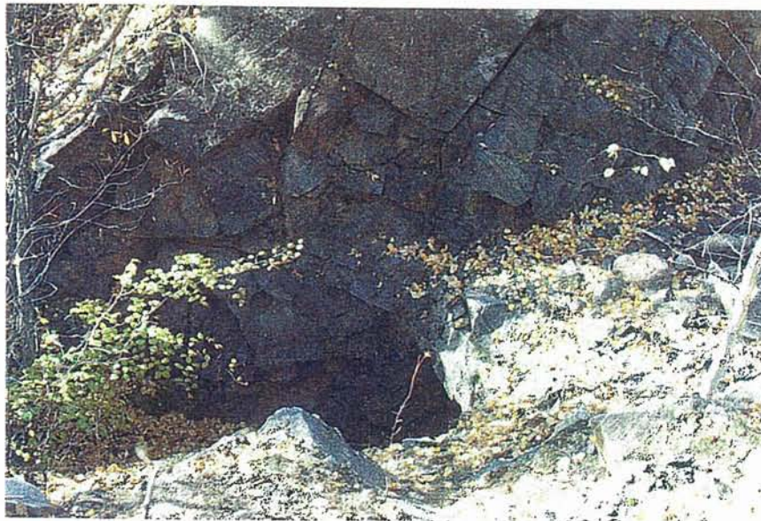
Photo 6.9-2 Consolidated Beta Gamma Shaft Opening; Note Bridge of Rock Between Shaft and Breakthrough to Surface on Left of Photo September 29, 2001
