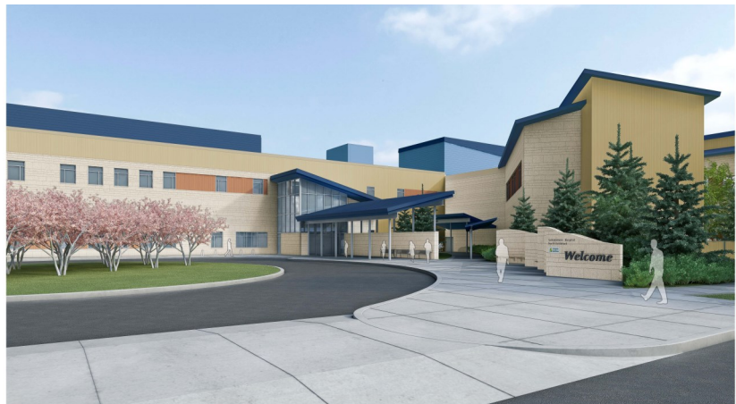
Main Entrance - Exterior
