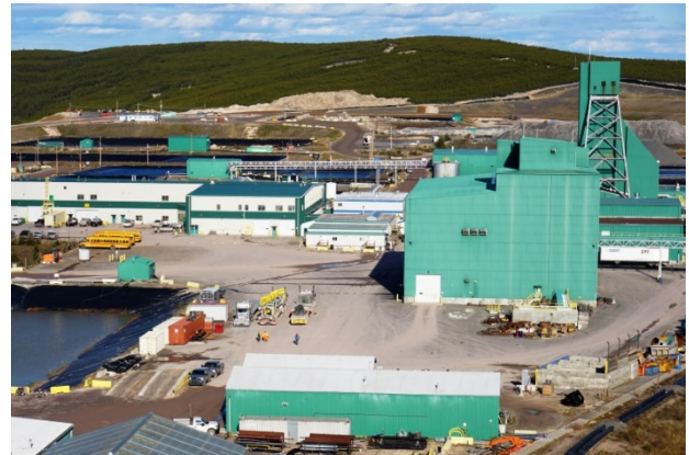
The McArthur River mine site is compact, occupying an area of approximately one square kilometer of leased Crown land.
