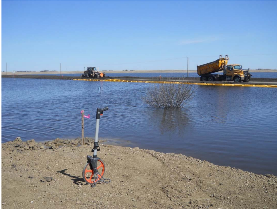
Figure 13.12 Highway No. 6 south of the Town of Southey with construction of shoulder berms (Photo Source: Walker Projects Inc. Spring 2015)
