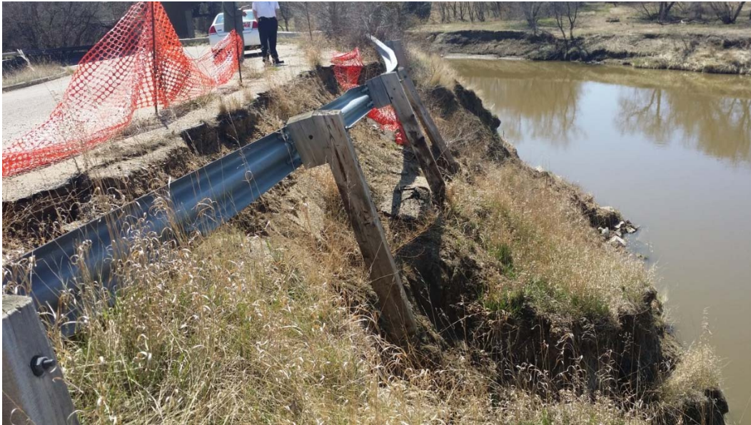
Figure 13.2 Slope is extremely unstable, 12 m drop into the river
