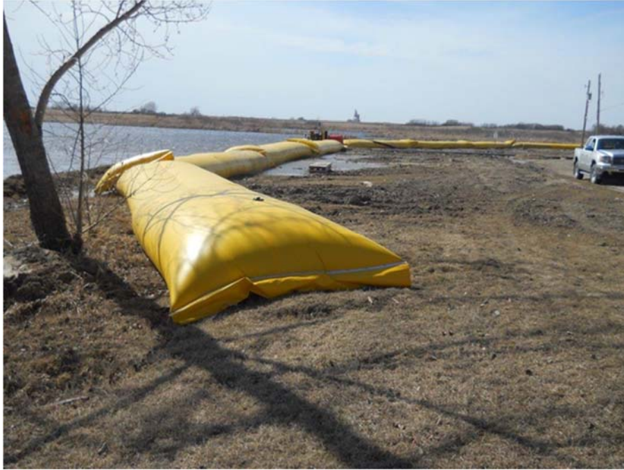
Figure 13.14 Town of Southey, Lions Park and Campground, Water Berms and Pump (Photo Source: Walker Projects Inc. Spring 2015)
