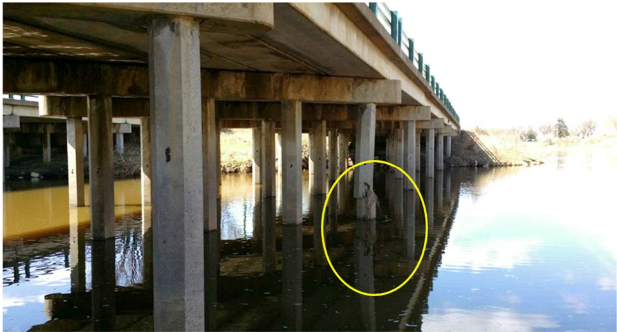
Figure 13.4 Ice flow damage to the concrete pillar on Manitoba Expressway
