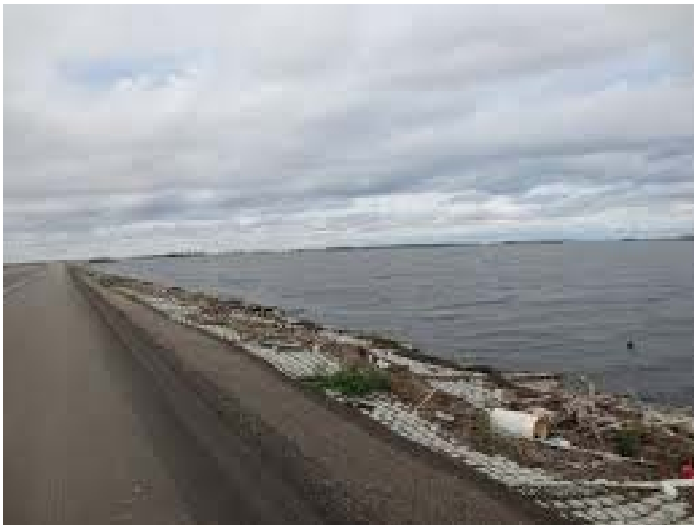
Figure 13.28 Highway 6 near Dafoe; 1-km section of road was raised, and shoulders were armoured to protect against wind and wave erosion.
