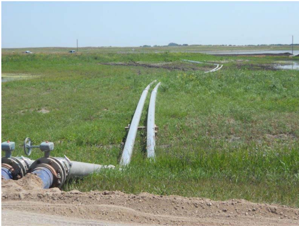
Figure 13.17 Relief pump lines taking flood water from Southey Basin to Loon Creek (about 12 km) (Photo Source: Walker Projects Inc. Summer 2015)
