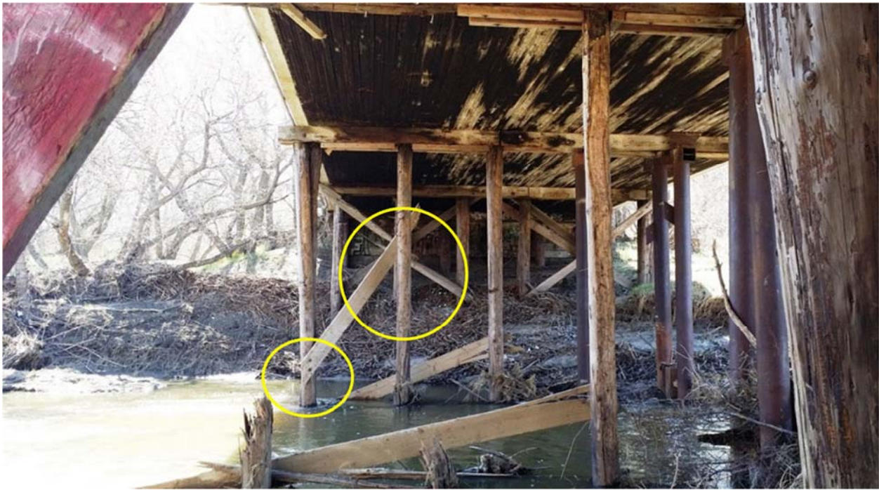
Figure 13.6 Broken piles and cross bracing; the ones that are still in situ are severely damaged and need to be replaced
