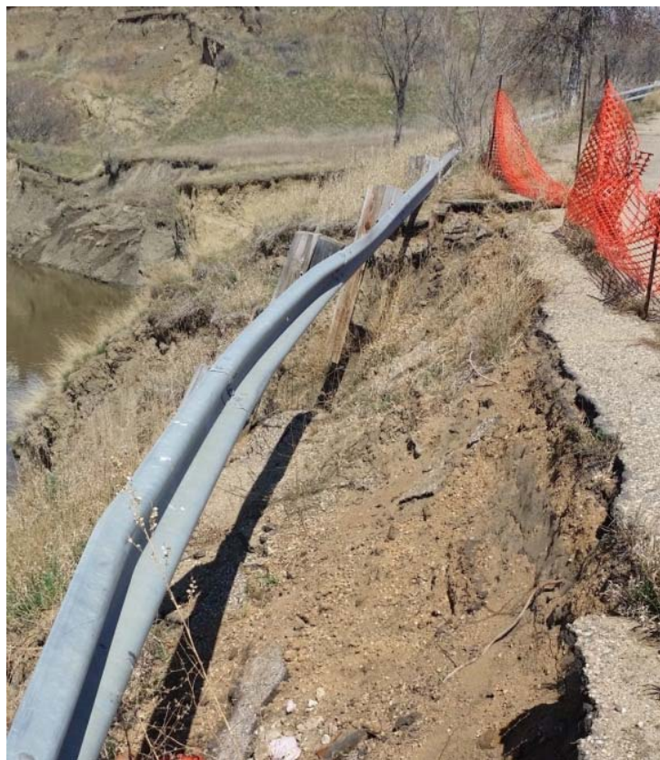
Figure 13.3 Road and side slope failure
